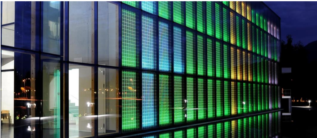
Ertext Solar – BIPV-Facade with LED, Fondation Pierre Arnault, Architect: Jean Pierre Emery
