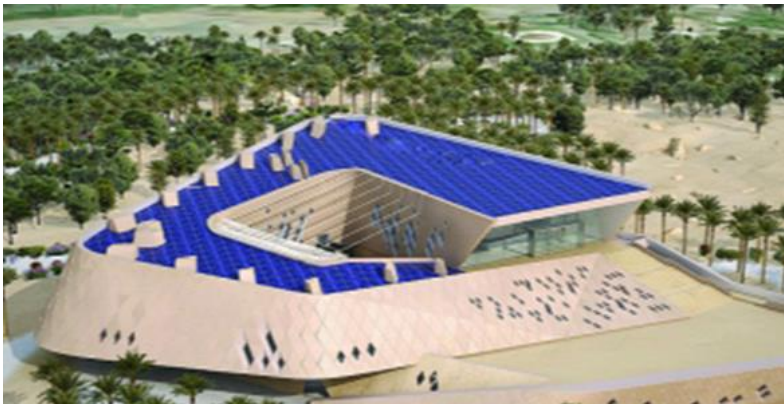
PV-Roof as major energy source Sheik Desert Centre
